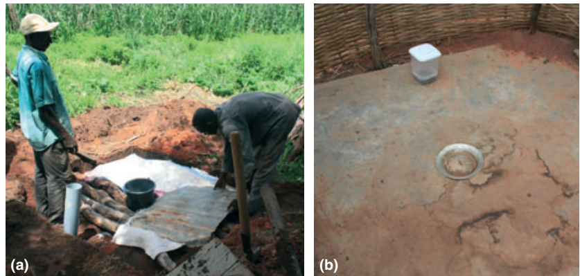
Figure 1 Construction of a latrine flytrap. (a) Here, a membrane is applied over a row of logs before concreting. In the centre is the bucket acting as a mould for the drop hole and to the left is the vent pipe on which the trap is positioned. (b) The completed latrine with drop hole cover and flytrap in place.
